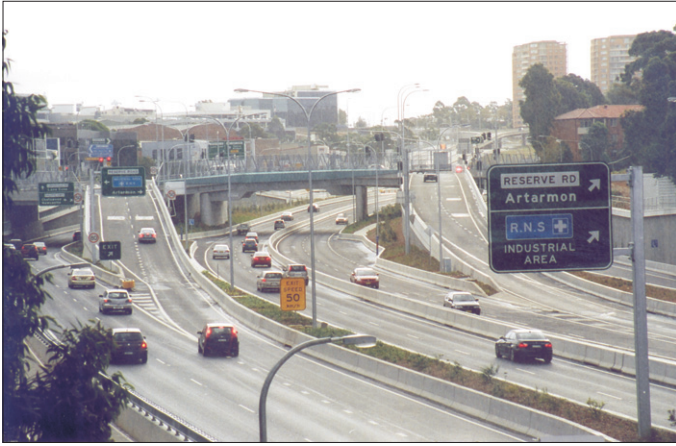
Looking west along the widened and reconfigured Gore Hill Freeway at the rebuilt Reserve Road overpass in Artarmon, 25 March 2007.
