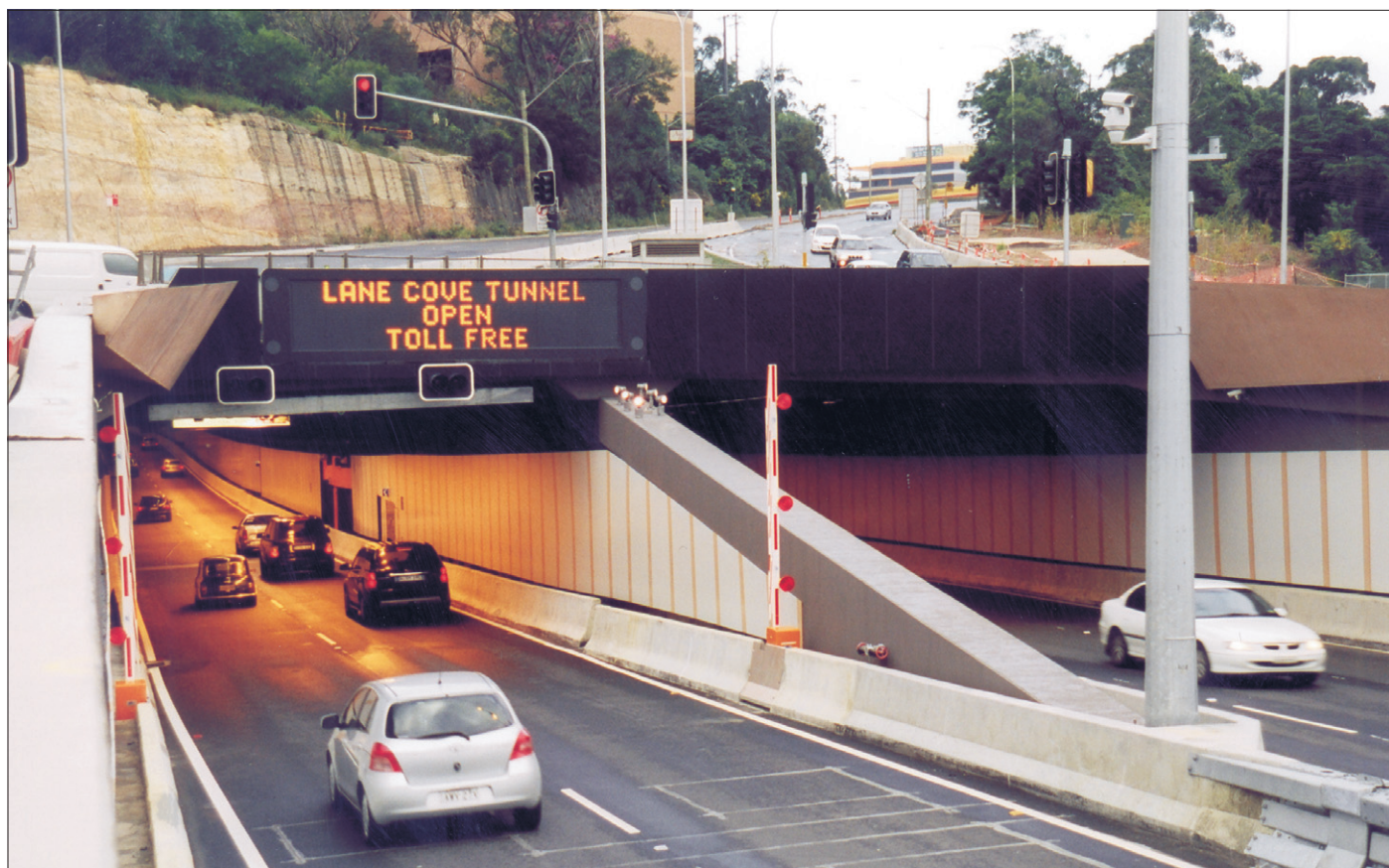
The western portals of the Lane Cove Tunnel, at the junction of Epping Road and Mowbray Road West in Lane Cove, on the day the tunnels opened, 25 March 2007.
