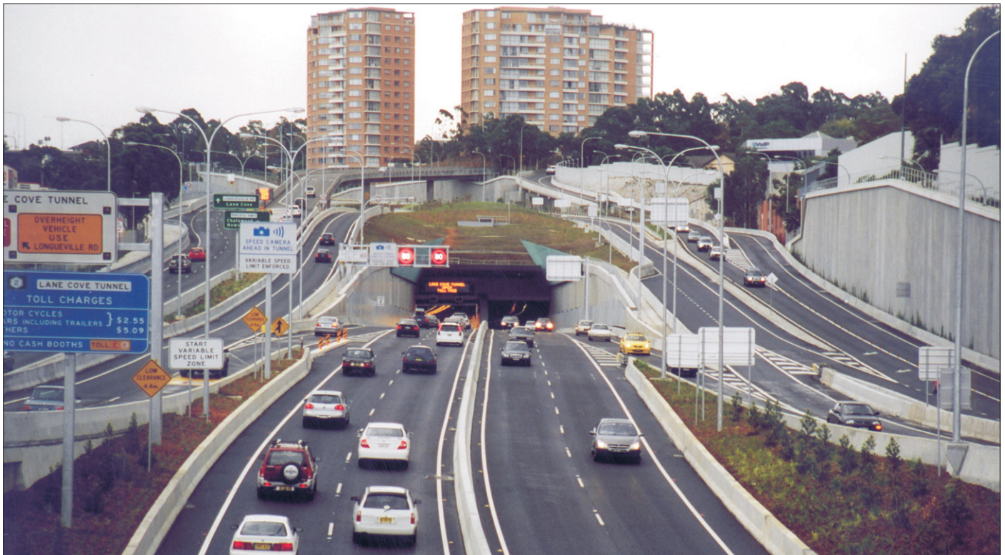
Looking west from the rebuilt Reserve Road bridge over the Gore Hill Freeway in Artarmon towards the eastern portals of the Lane Cove Tunnel, 25 March 2007.
