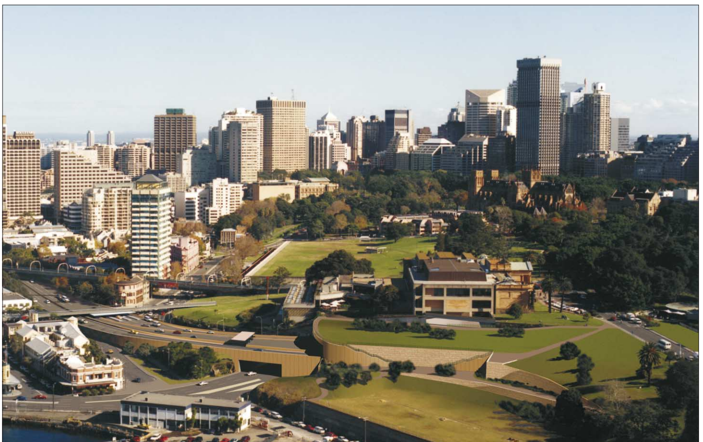
Artist's impression of the main toll plaza and the landscaped canopy being built over the Eastern Distributor next to the Art Gallery
